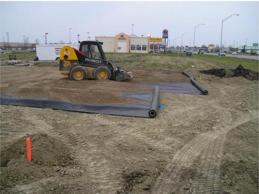
The soils engineer might recommend placing several inches of clean "crushed" material (DOT base course) in the floor area this fall for the purpose of bridging over the soft silty soils next spring. Sometimes, a heavy duty geotextile fabric can also be placed to help reduce the thickness of "crushed" material that is needed. These are probably unanticipated costs, but they may be cheaper than drying or replacing 1-2 feet of muddy soils in an enclosed building during early spring.
