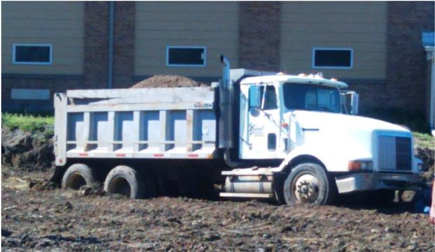
Come March, the building is heated and WOW, the floor area turns into a big mud hole!!! The top two feet of soils is nothing but mush. How could this happen... loaded trucks were driving on it last fall? Now, skid loaders are having a tough time getting around, let alone trucks that need to place the final 6" of sand and then the concrete floor. Worse yet, the
